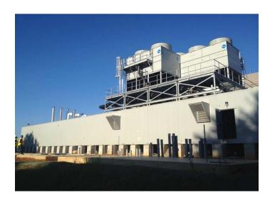
Holy Cross Germantown Hospital needed a solution that maximized the allowable area of the building, provided very high quality mechanical components and offered maximum efficiency. The solution involved the incorporation of an Epsilon packaged mechanical plant. This is a free-standing, completely factory designed, engineered, and fabricated mechanical plant. It consists of boilers, chillers, pumps, cooling towers, and electrical system.
